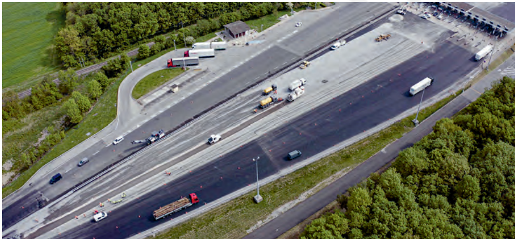
© Eiffage Route Centre Est
