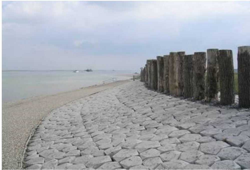
Example of coast protection design used in France
